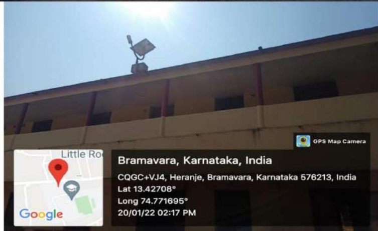
Solar Energy Lights
