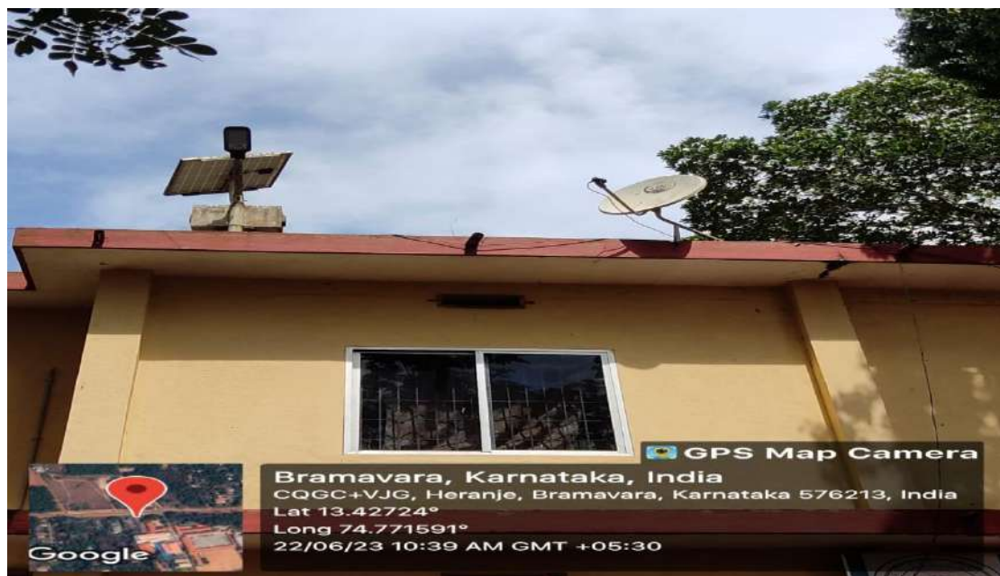
Solar Energy Lights
